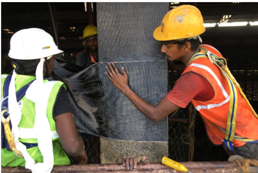
View of CFRP Wrapping.
