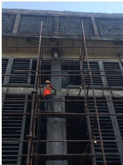
View of Polymer modified mortar application
