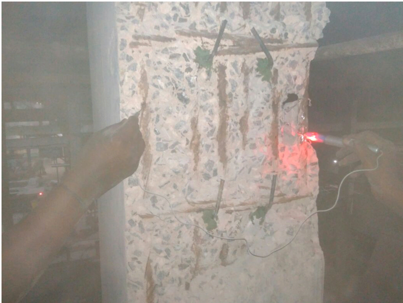
View of sacrificial anode Galvashield installed and connectivity checking
