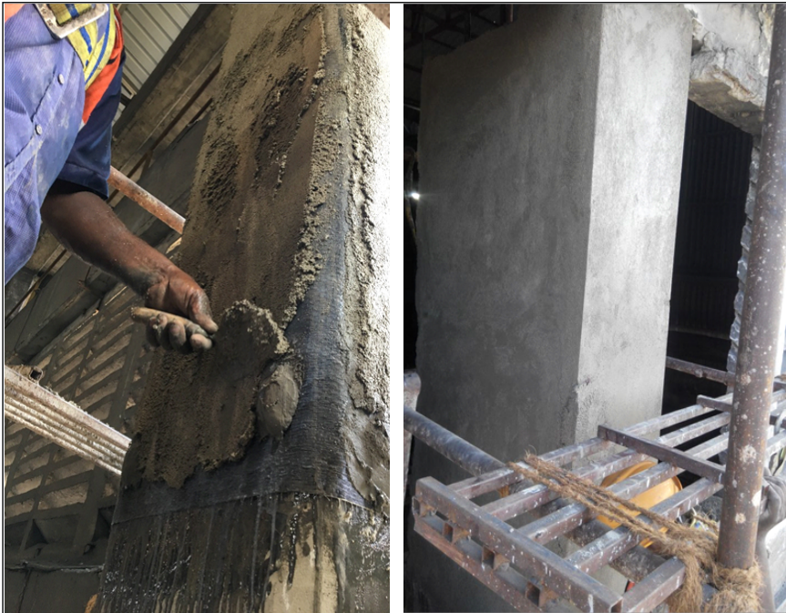
Application of Sinicon PP over CFRP and the finished view
